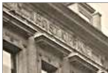
Figure 7: Close-up of “ POST OFFICE ” stone façade.
