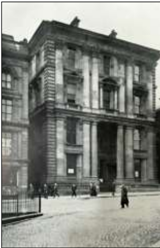
Figure 4: photo of Post Office building (circa: 1900 ).
