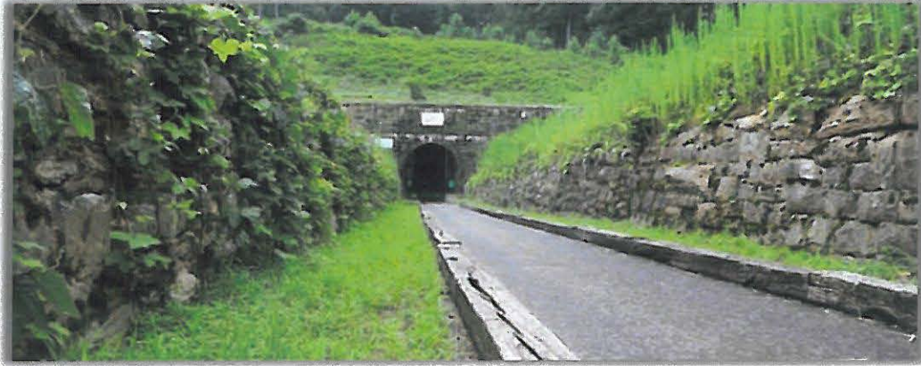
Figure 5. Contemporary view of Chetogeta Mountain tunnel.
