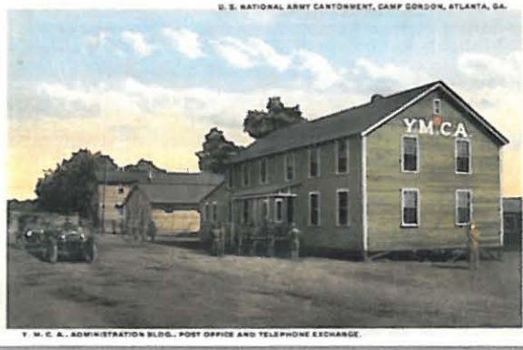
Figure 12. Camp Gordon YMCA facilities.
