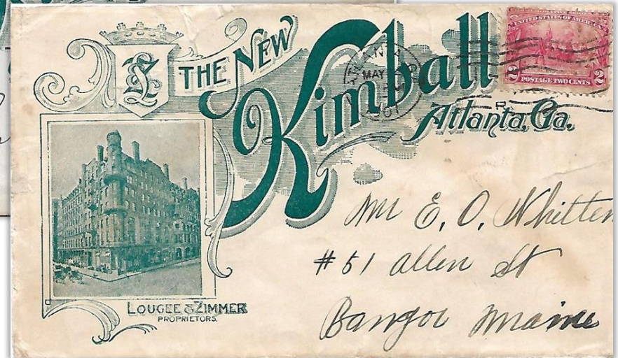
Figure 8. The New Kimball, Atlanta.
